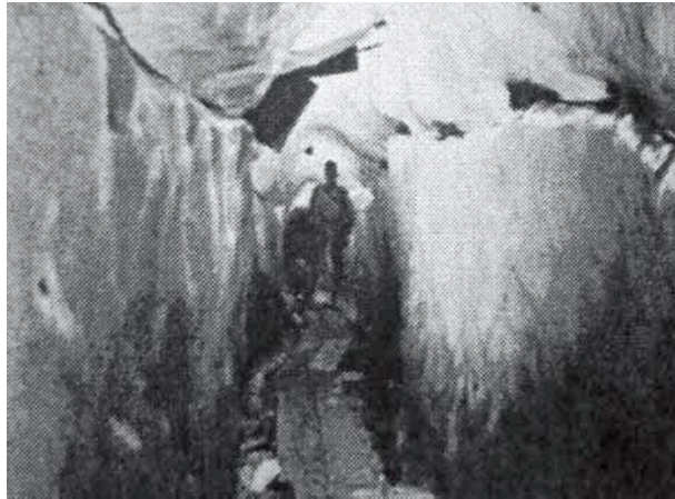
Fig. 2 - Exemption of tunnel excavated in ice (Brescia C.A.I Archives).
